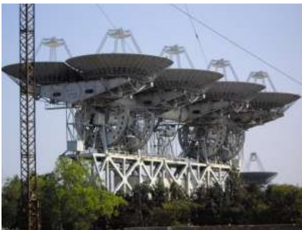
Fig. 3 A Pluton receiver antenna with eight 16m duralumin parabolic dishes
