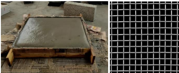
Fig 3.2. Casting of Slab – I
