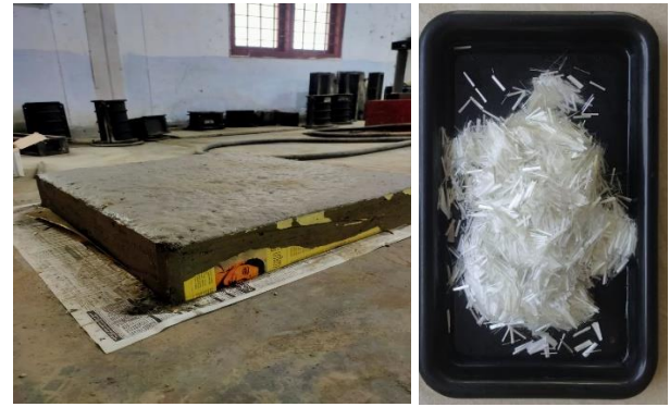
Fig 3.3. Casting of Slab – II
