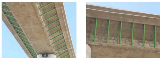
Fig 1. Tubular columns in bridges
